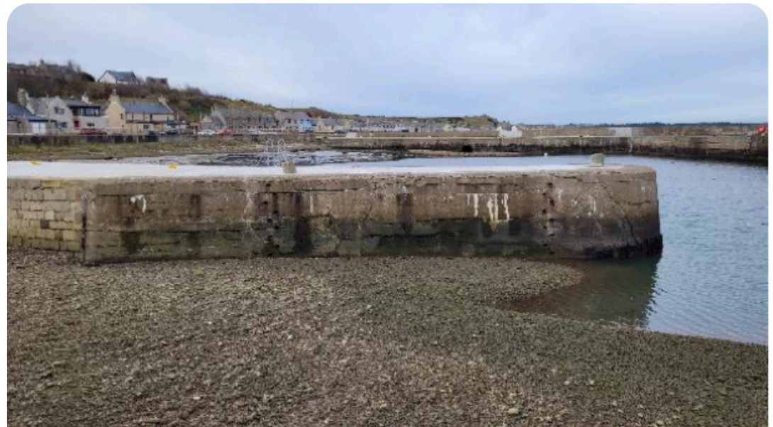
Photo 49: Middle Pier – East side
